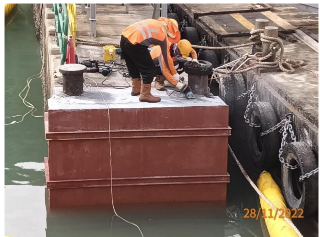
Removal of two bollards
