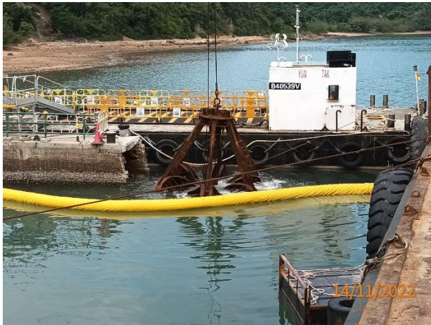
Removal of Broken Concrete Pieces
