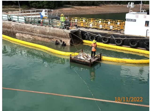
Repair Works at Catwalk by Installation of Bagged Concrete
