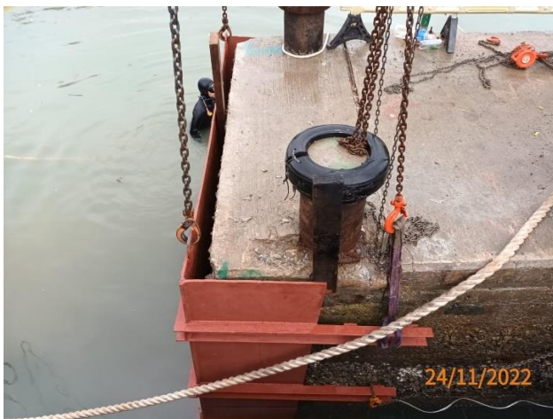
Repair Works at Pier Head by Installation of Steel Plates
