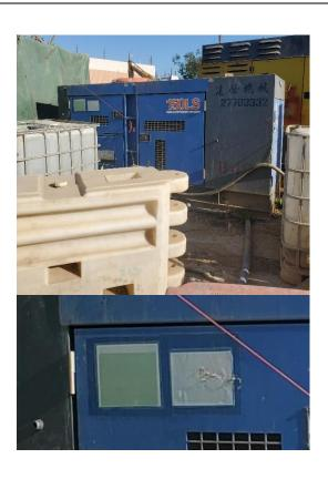
Reminder 1: The unclear NRMM label and QPME label of the generator should be replaced
