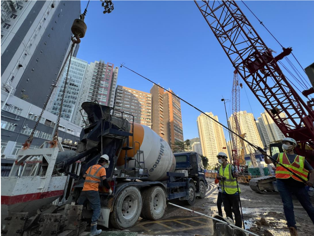
Photo C2. Measurement Photo for Concrete Discharge Mode
