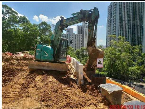
Construction activities: Backfill
