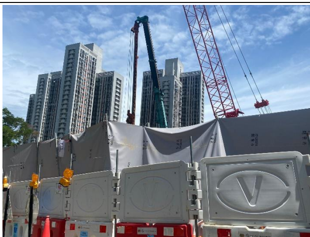
Mitigation Measures: Noise barriers were erected during the construction works
