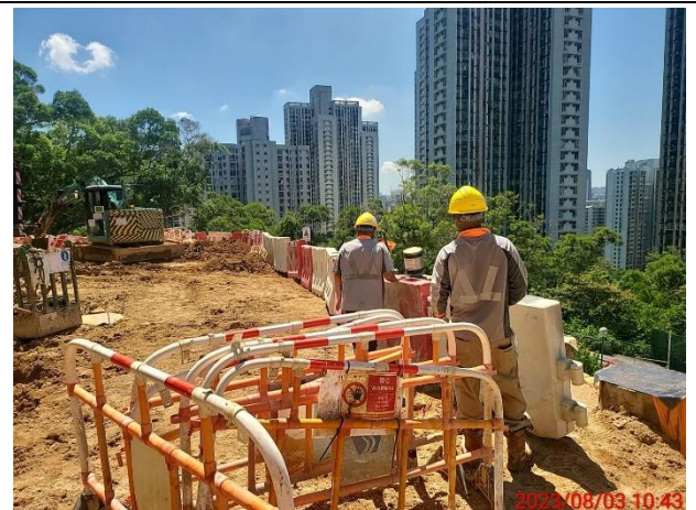
Construction activities: Setup water-barrier and housekeeping
