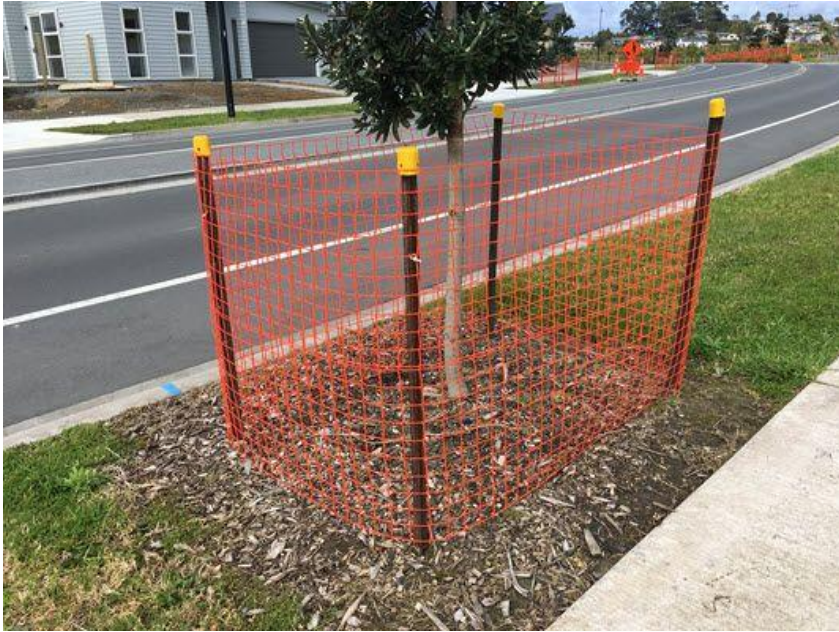
Similar Type of Temporary protective net/fencing that will be provided at P2, P3 and P6
