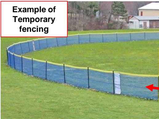
The temporary fencing should have at least 0.5m in height and no hole for animal to pass.
