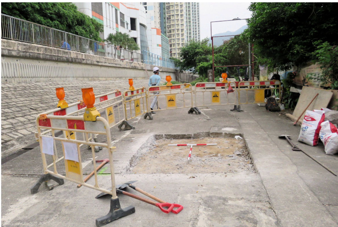
Plate 18 General view of TP3 area, looking south
