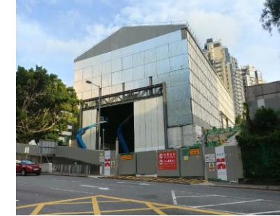
Photo E3.1: Sample Photos of Noise Enclosure (Central Kowloon Route – Central Tunnel)
