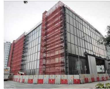
Photo E3.1: Sample Photos of Noise Enclosure (Central Kowloon Route – Central Tunnel)
