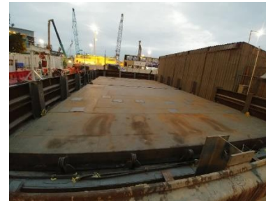
Photo E3.2: Sample Photos of Noise Cover (Central Kowloon Route – Central Tunnel)
