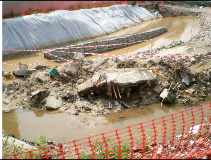
The C&D waste along the slope was reminded to remove to improve house-keeping on the site. (MUP04)
