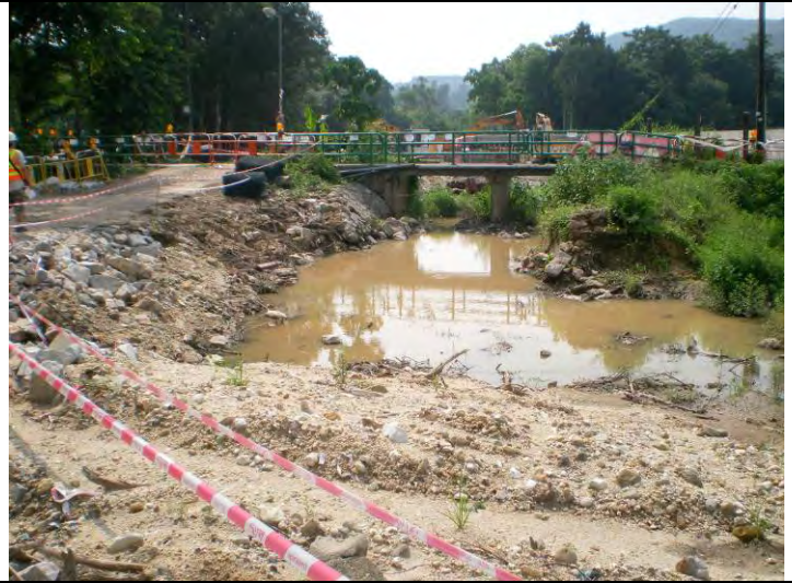
The stagnant water accumulated should be drained away or applied larvicidal oil to prevent mosquitoes breeding. (MUP05)
