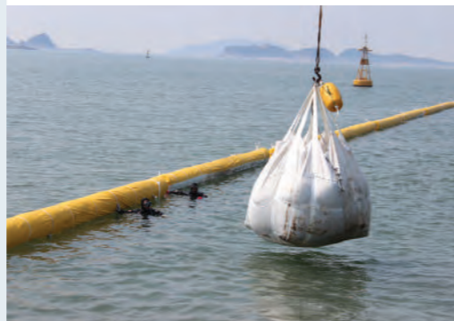
GEONIA® Ton Bag Anchor being installed
