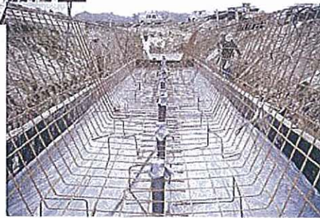
Channel of Drainage 河道骨架
