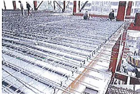
Floor Making of Buildings 多層大廈之樓面鋪設
