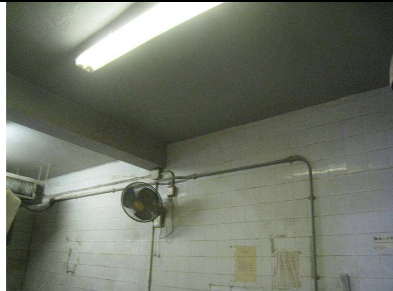
Description: Existing Condition of the Storage Room under Cremation Room 2 (CR2)
