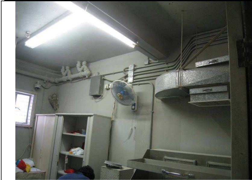
Description: Existing Condition of the Storage Room under Cremation Room 2 (CR2)
