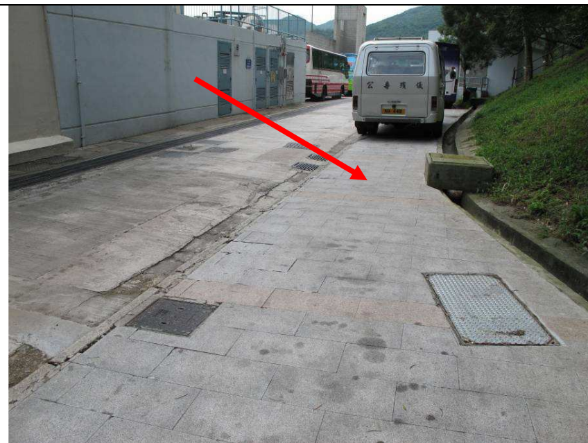
Description: Location: Trial Pit 1(TP1)
