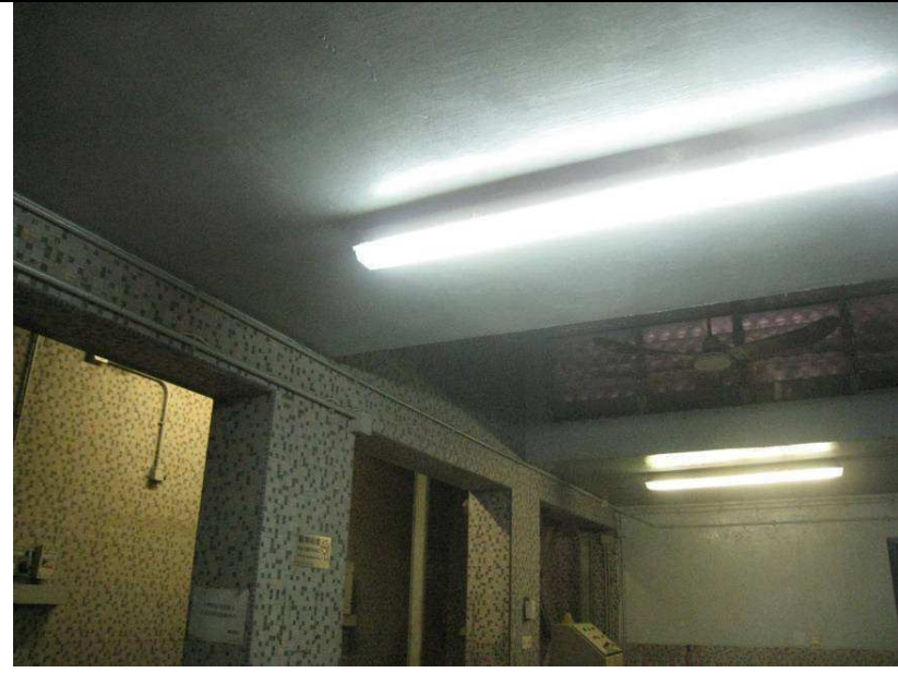
Description: Existing Condition of the Storage Room under Cremation Room 1 (CR1)
