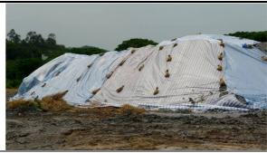
Capping of the PFA has been established on site to prevent spreading in the air.
