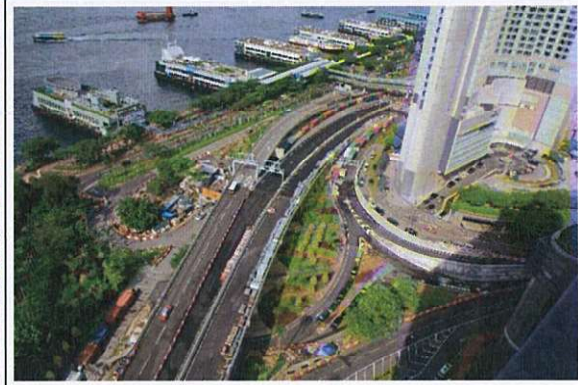
V10 - Connaught Road Central Flyover (near Four Seasons Hotel)
