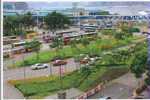
V4 - Man Yiu Street Bus Terminus (view from IFC Mall)
