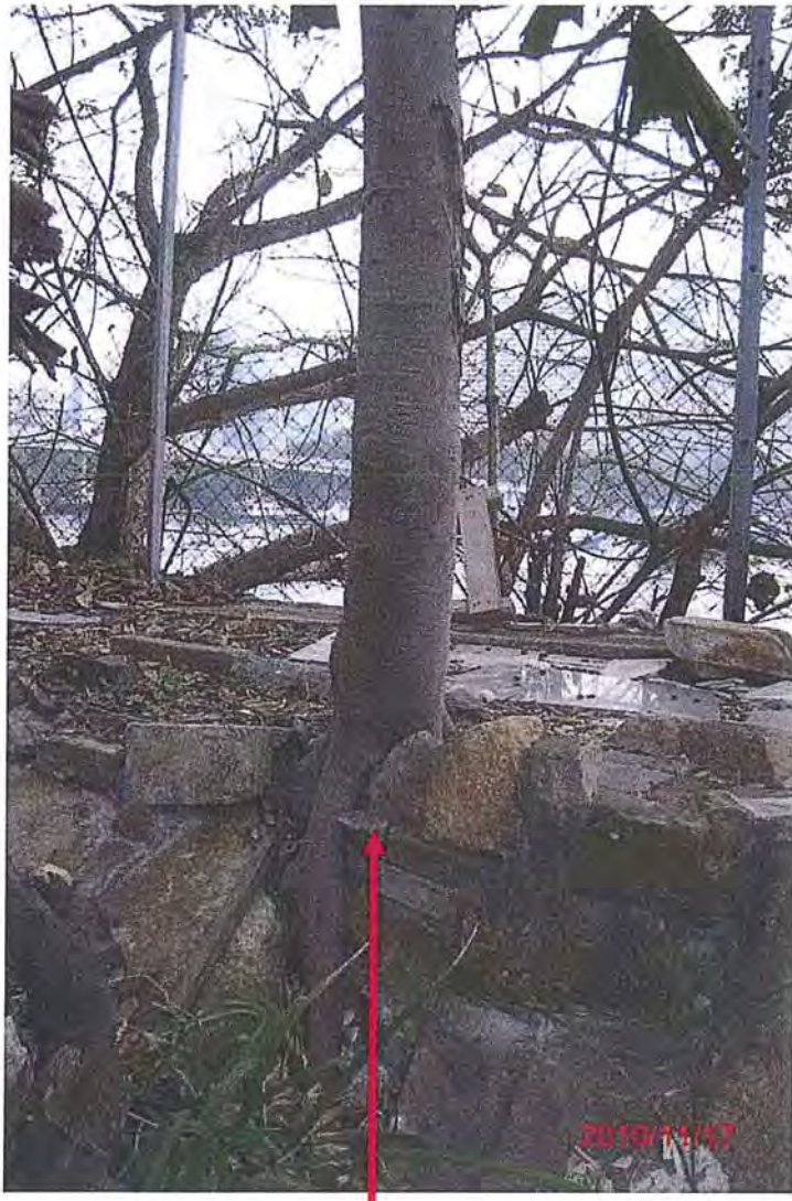
Root system distorted due to rock. Limited root system coverage for stability.
