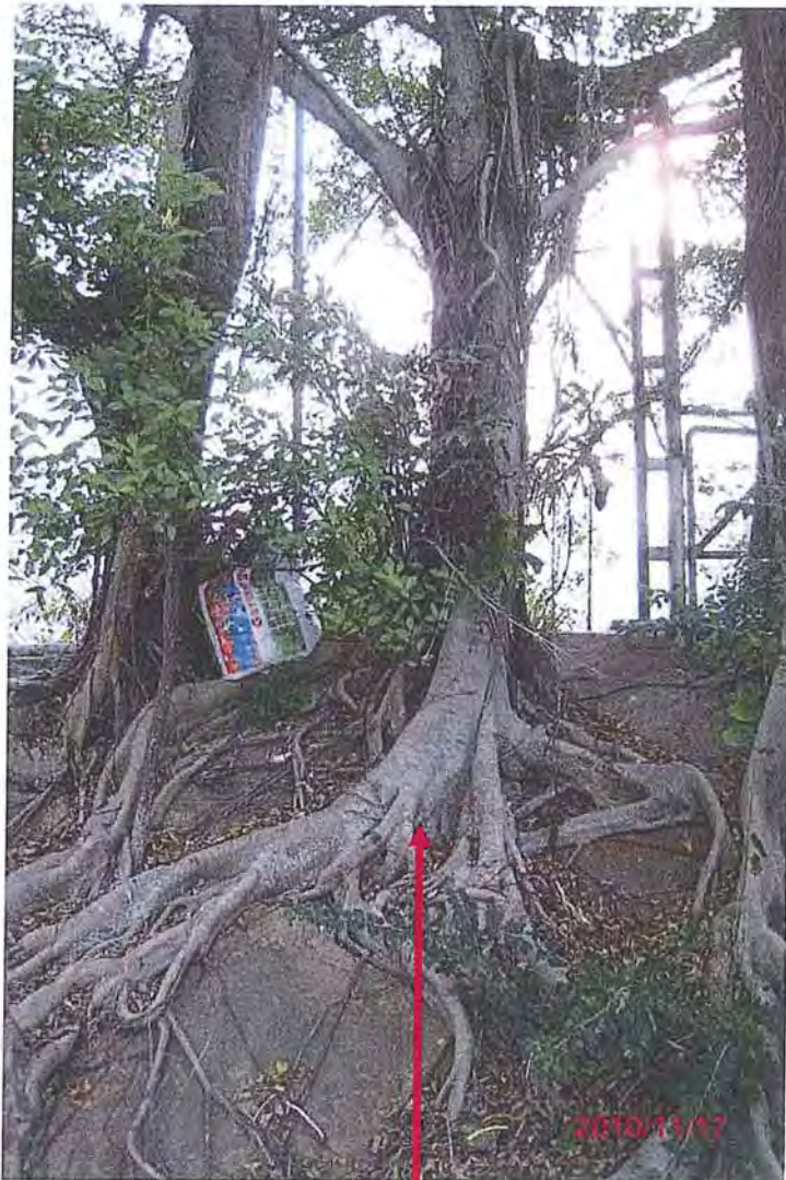
Rootball locates on large boulder at slope and clashing with adjacent roots of trees. Preparation would drastically affect rootball and structural stability
