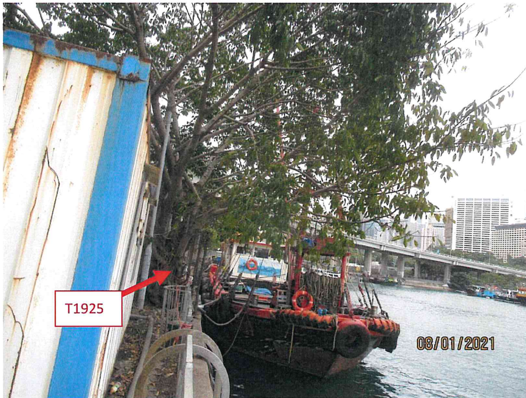
The pier may be open to public after the site office removed this year. Follow-up action on T1925 will be considered to be taken.
