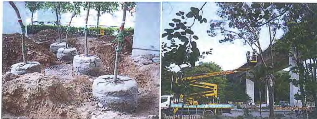
Tree Transplanting works - Wideneing of Tolo Highway NT
