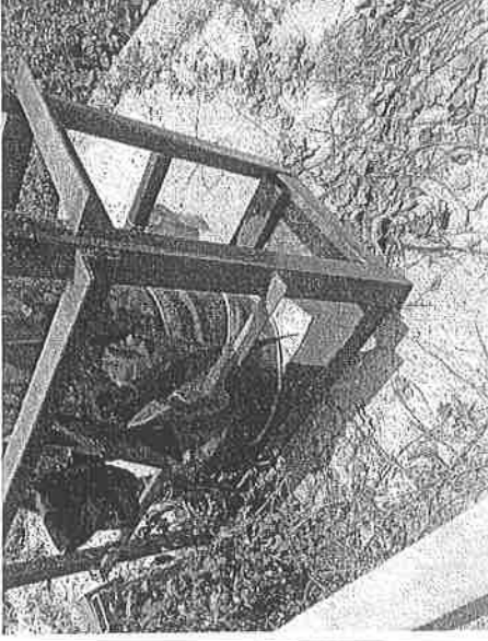
Photo 140528_001 – Water pump was provided for draining down the stagnant water near the middle section of New Road site.
