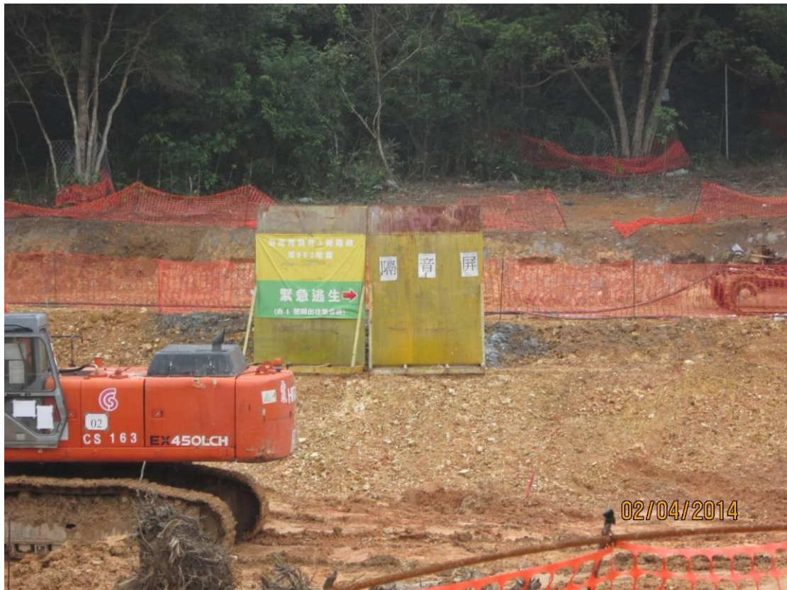
Fig. 2 –The noise barriers were provided for soil nail activities to minimize the noise impact.
