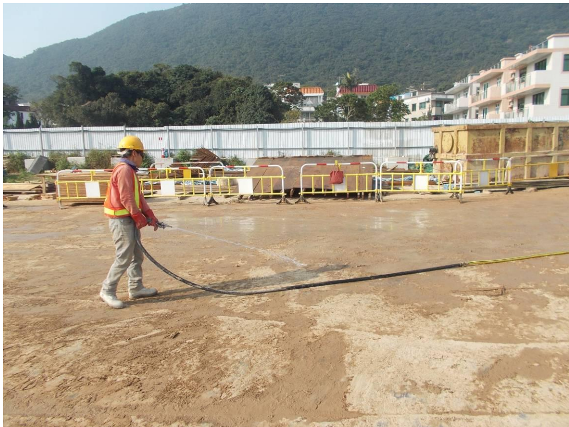
Fig.4 –Water spraying was provided by frontline staff for dust suppression.
