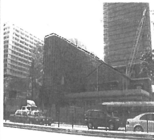
Temporary Noise Barrier Screening Noise to Sensitive Receivers (Former Marine Police Headquarter, TST)
