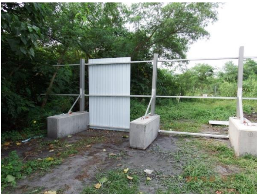
Installation of site hoarding
