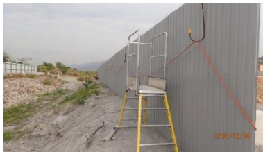
Improvement of site hoarding
