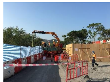
Removal works of asbestos pipe
