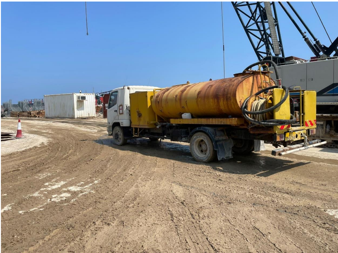
Figure 7: Photo Record of Using Water Bowser to Water Main Haul Road
