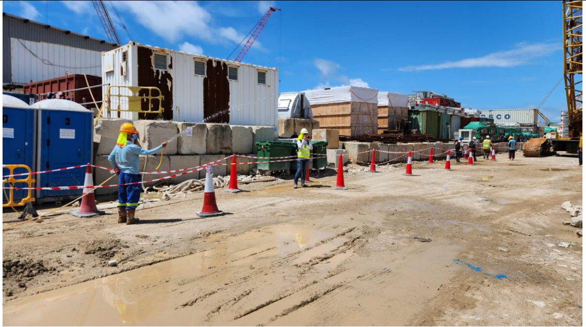
Figure 10: Photo Record of Spraying Water to Main Haul Road
