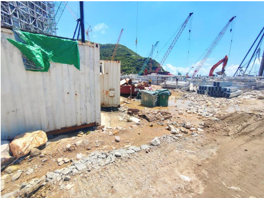
Figure 5: Site Photo of Main Haul Road Taken during Site Inspection on 19 June 2023
