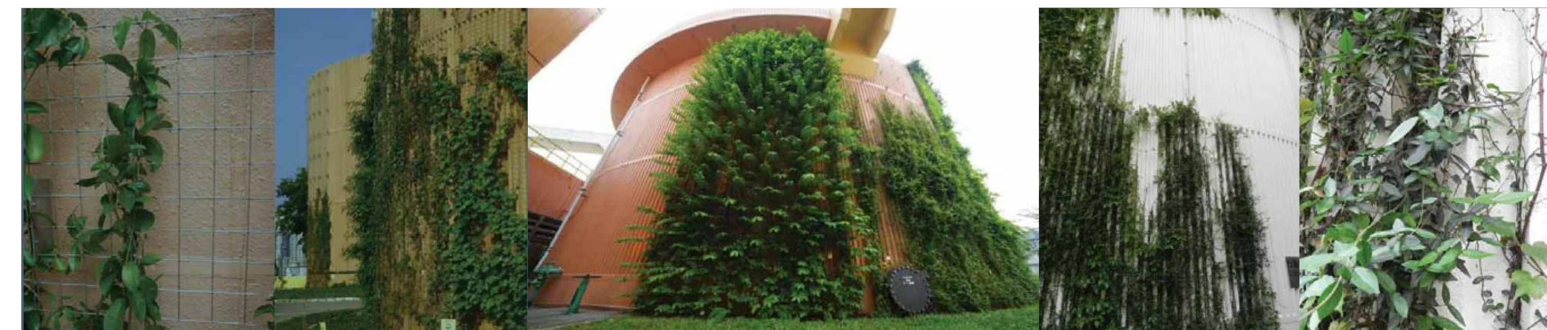
VERTICAL GREENERY REFERENCE IMAGE OF Pseudocalymma alliaceum IN SHA TIN SEWAGE TREATMENT PLANT
