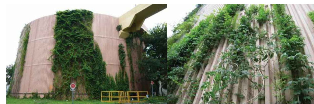
VERTICAL GREENERY REFERENCE IMAGE OF Bauhinia corymbosa IN SHA TIN SEWAGE TREATMENT PLANT VERTICAL GREENERY REFERENCE IMAGE OF Campsis grandiflora IN SHA TIN SEWAGE TREATMENT PLANT
