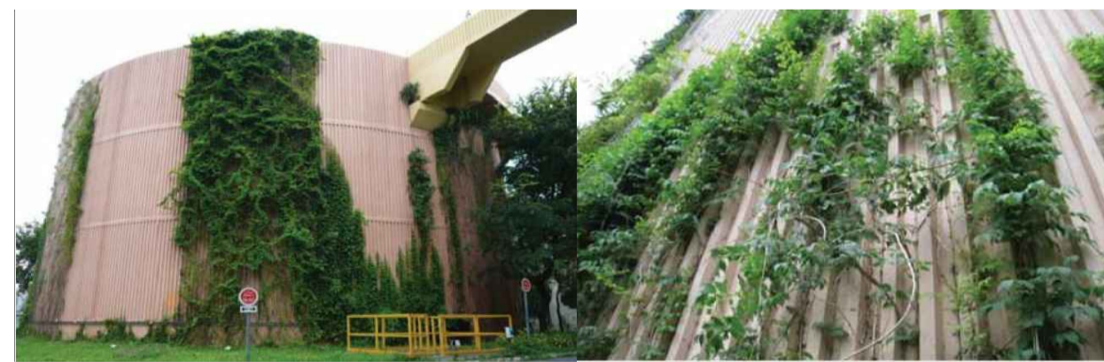
VERTICAL GREENERY REFERENCE IMAGE OF Bauhinia corymbosa IN SHA TIN SEWAGE TREATMENT PLANT
