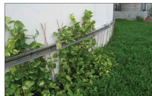
VERTICAL GREENERY REFERENCE IMAGE OF Epipremnum aureum IN SHA TIN SEWAGE TREATMENT PLANT
