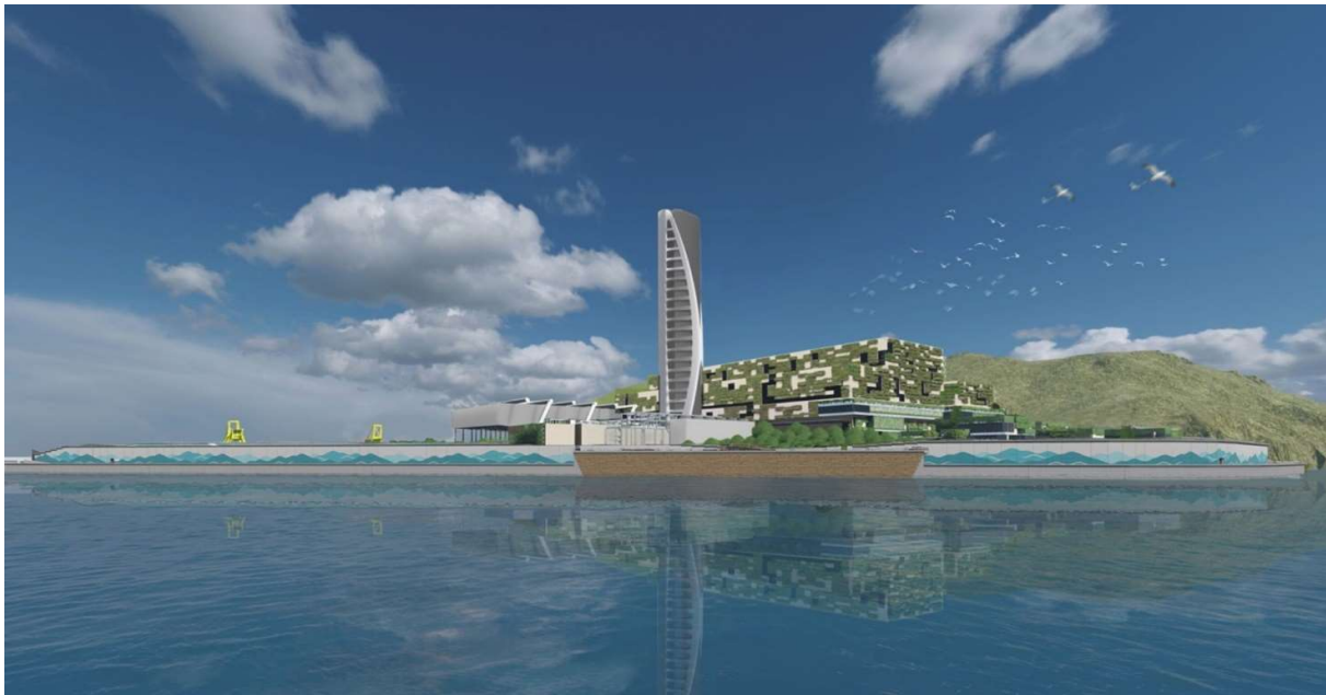
Figure 6.1 General Aesthetic treatment of the IWMF development featuring the timber hull-like seawall/wavewall in the foreground, landscaped development with vertical greening in the midfield and the iconic sail format chimney structure.
