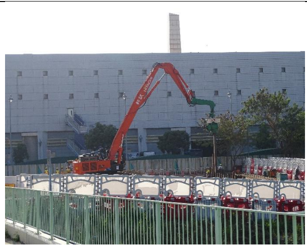
Vibration Hammer (Taken on 20 Jan 20)
