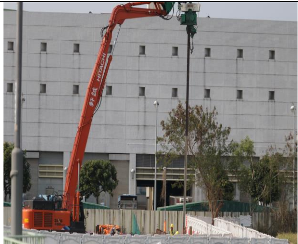
Vibration Hammer (Taken on 17 Feb 20)
