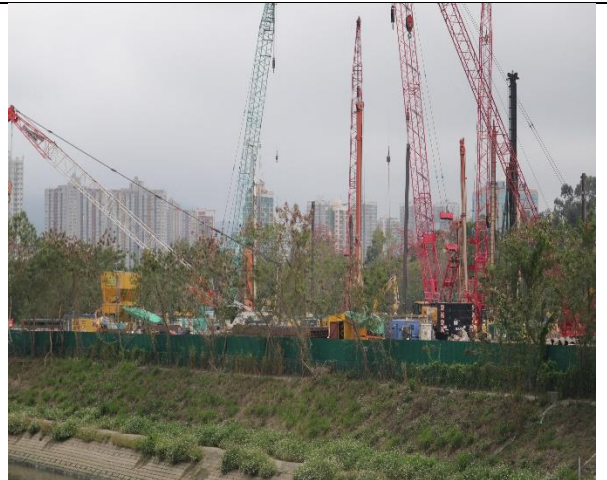
Vibration Hammer (Taken on 2 Mar 20)
