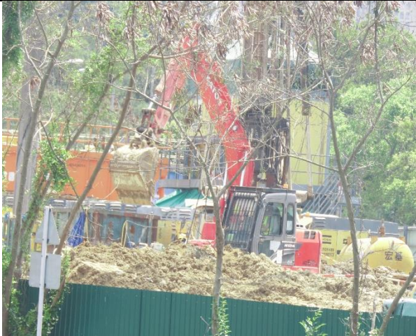
Excavation (Taken on 24 Mar 20)
