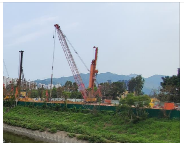
Vibration Hammer (Taken on 24 Apr 20)
