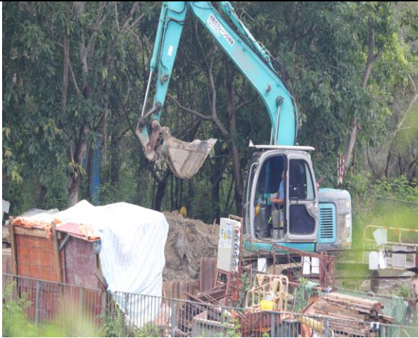
Excavation (Taken on 26 May 20)
