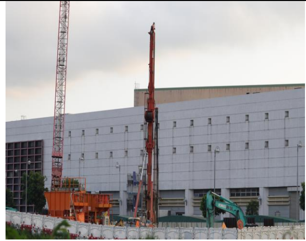
Sheet piling (Taken on 19 May 20)
