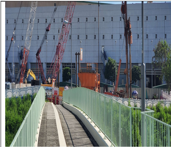
Excavation (Taken on 11 Jun 20)
