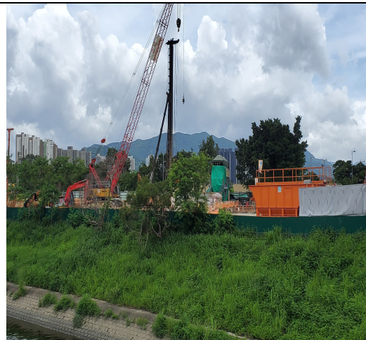
Vibration Hammering (Taken on 5 Jun 20)
