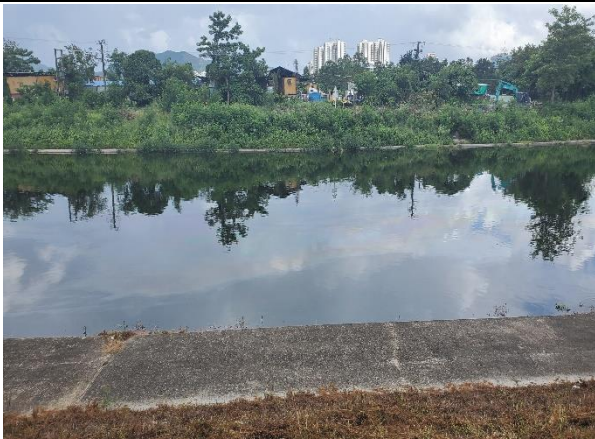
Oil stains (Taken on 7 Jul 20)
