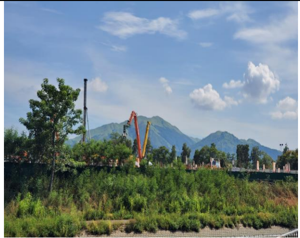
Vibration Hammer (Taken on 21 Jul 20)
