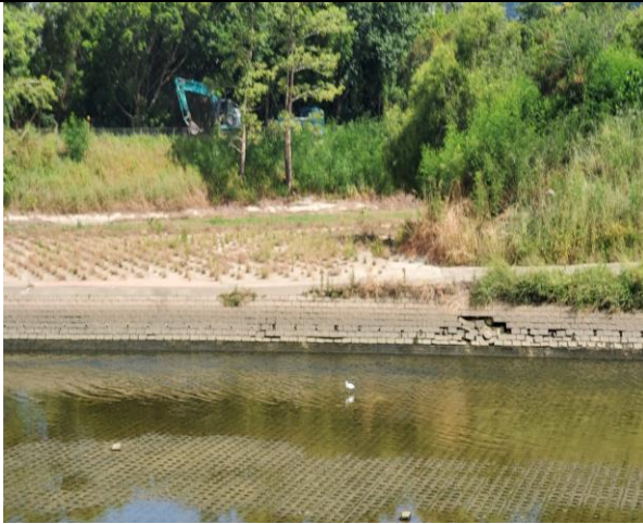
Excavation (Taken on 16 Jul 20)
