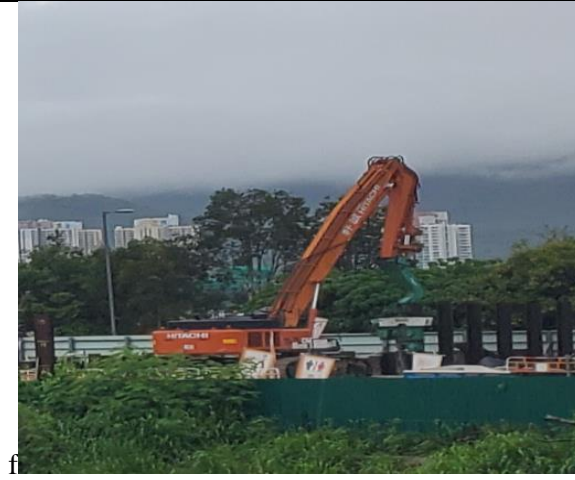
Sheet Piling (Taken on 28 Sep 20)
