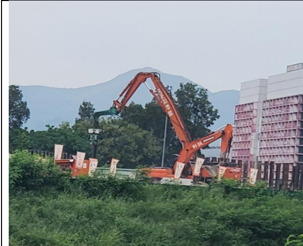
Excavation & breaking (Taken on 8 Sep 20)
