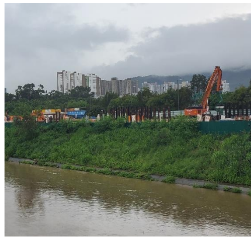
Excavation (Project-related, taken on 28 Oct 20)
