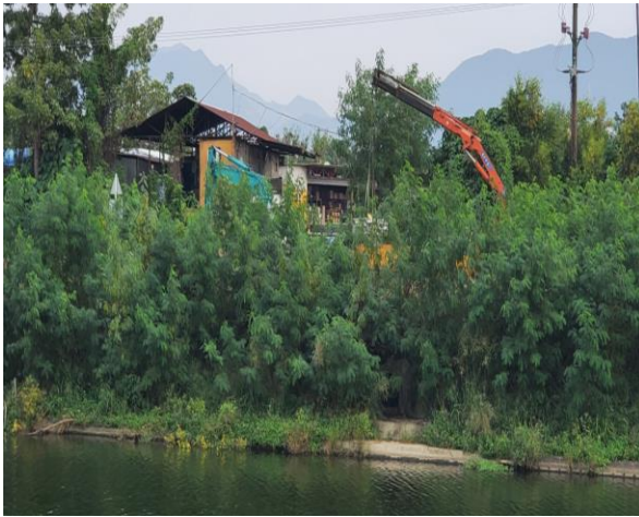
Excavation & Crane (Non project-related, taken on 20 Oct 20)
