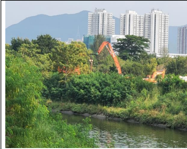
Sheet Piling (Taken on 16 Oct 20)
