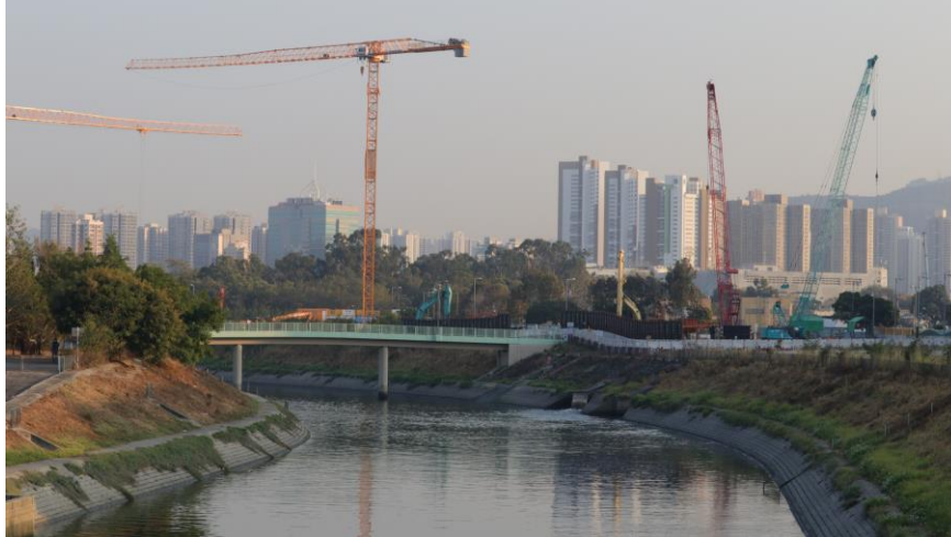
Excavation & Crane (Project-related, taken on 15 Jan 21)
