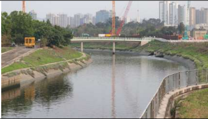
Excavation & Crane (Project-related, taken on 12 Mar 21)
