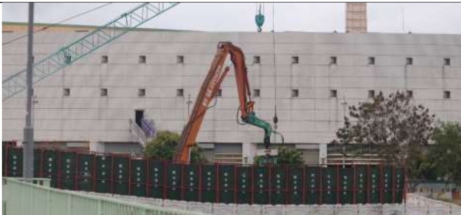
Sheet-piling (Project-related, taken on 29 Mar 21)
