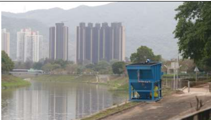
Placement of sedimentation tank (Non-project-related, taken on 29 Mar 21)
