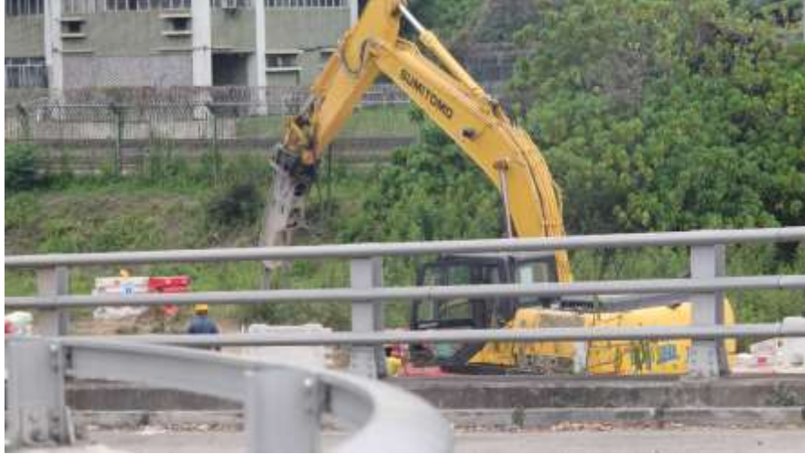
Breaking works (Non-project-related, taken on 29 Mar 21)
