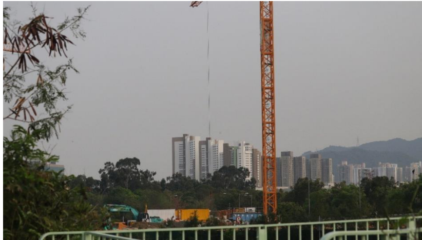
Excavation & Crane (Project-related, taken on 8 Apr 2021)
