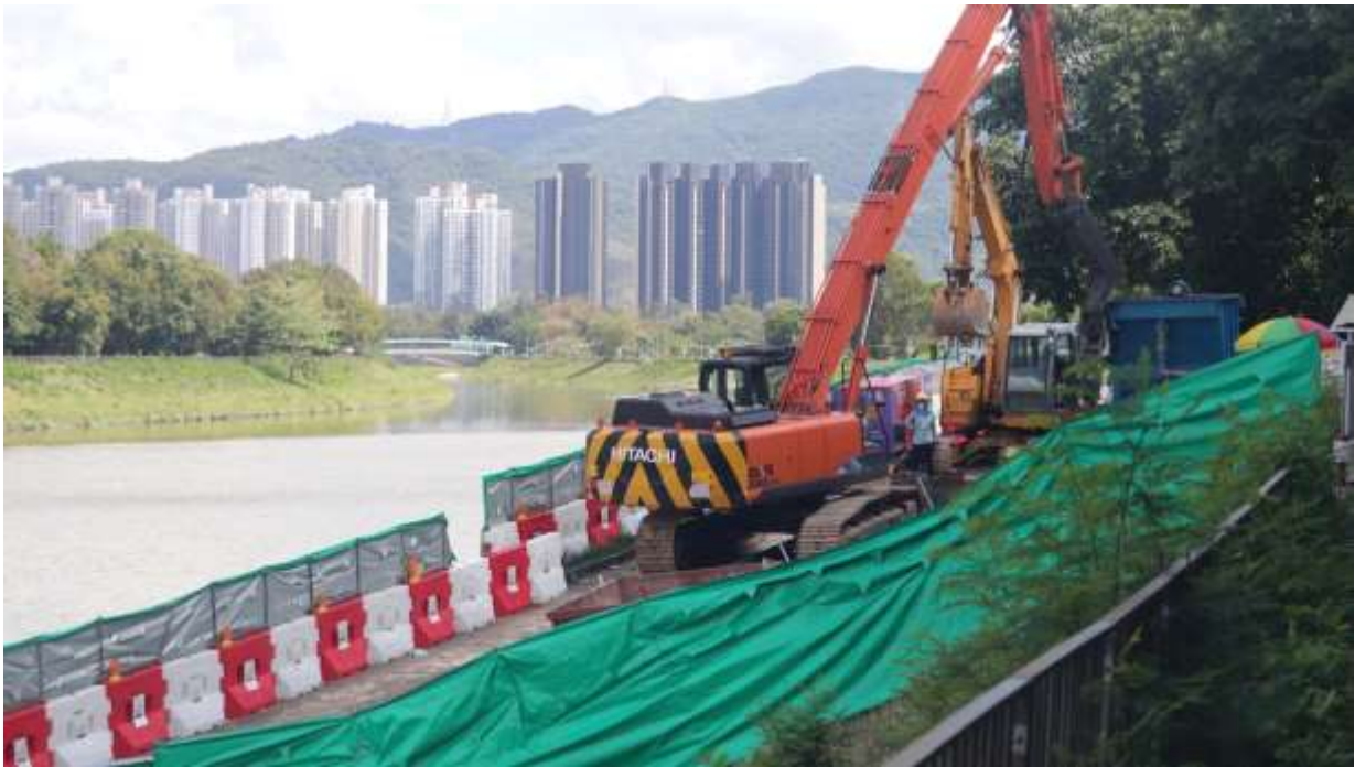
Sheet-piling, generator & welding works (Non-project-related, taken on 3 June 2021)
