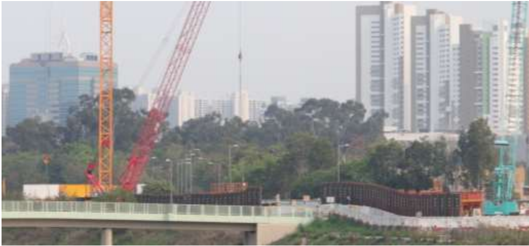
Excavation & Crane (Project-related, taken on 3 June 2021)
