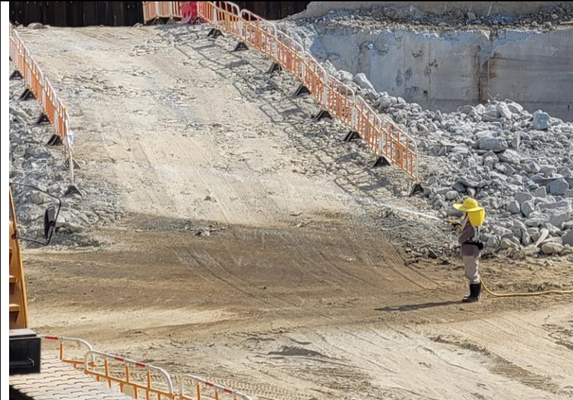
Water spraying method is adopted for minimizing dust generation.
