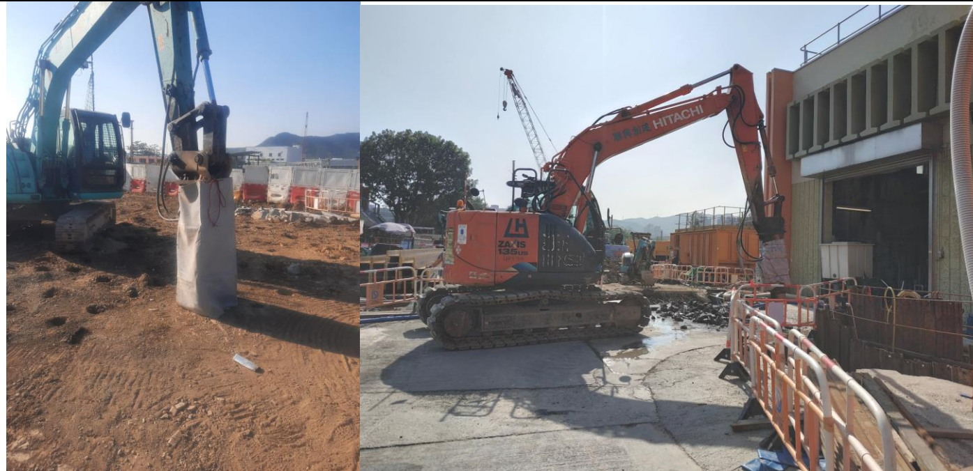
The breaking tips are covered with acoustic canvas
