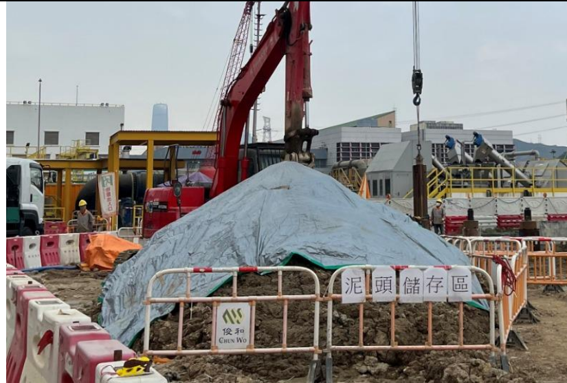
The stockpile is covered properly with tarpaulin.
