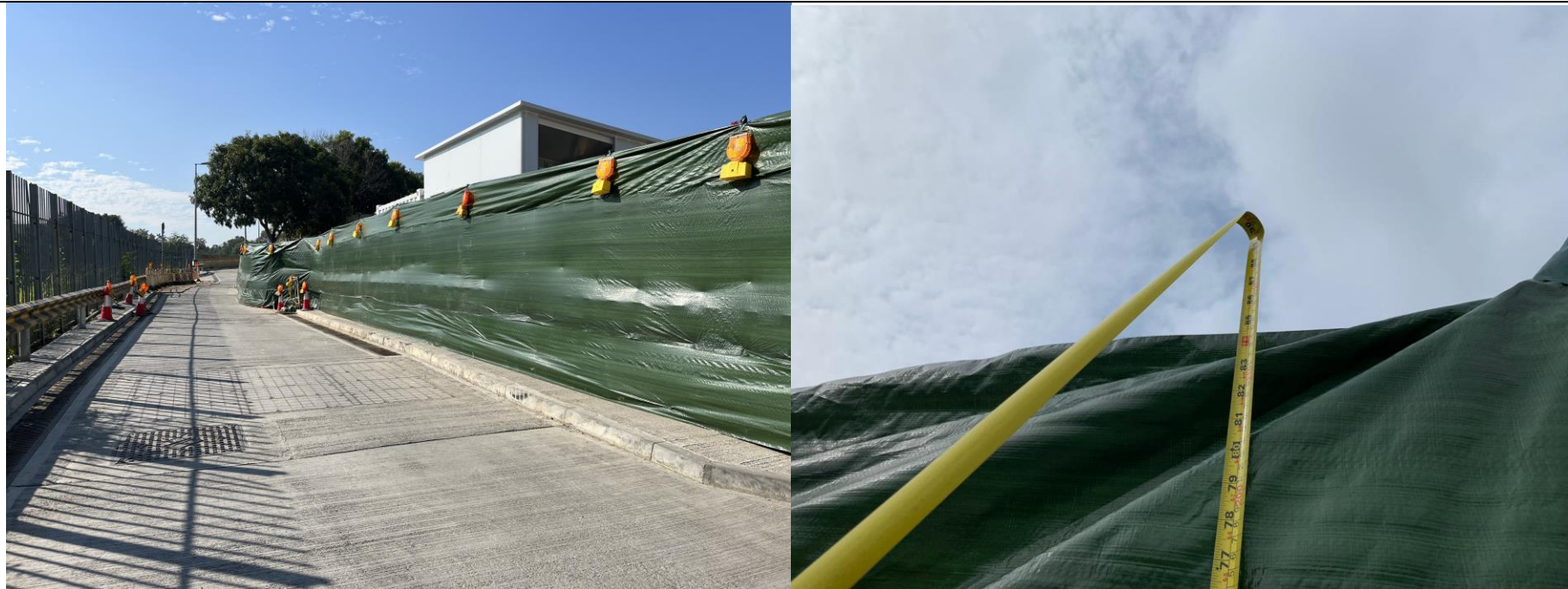
The site barrier next to Shek Sheung River (Sidestream) is completed
