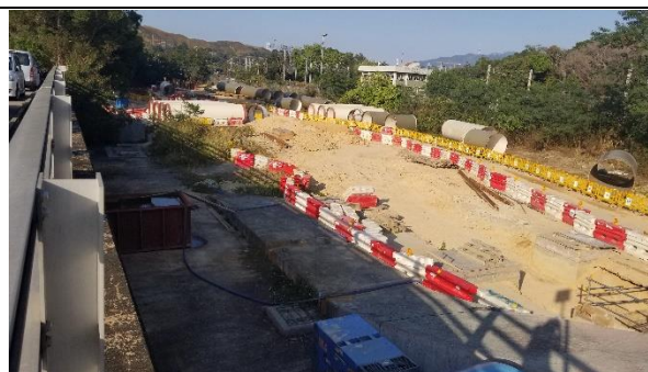
Construction Activities (Sheung Yue River) (Non-project-related, taken on 11 Feb 2022)
