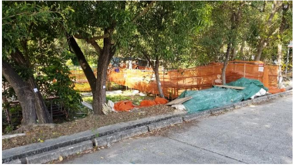
Construction Activities (Ng Tung River)
