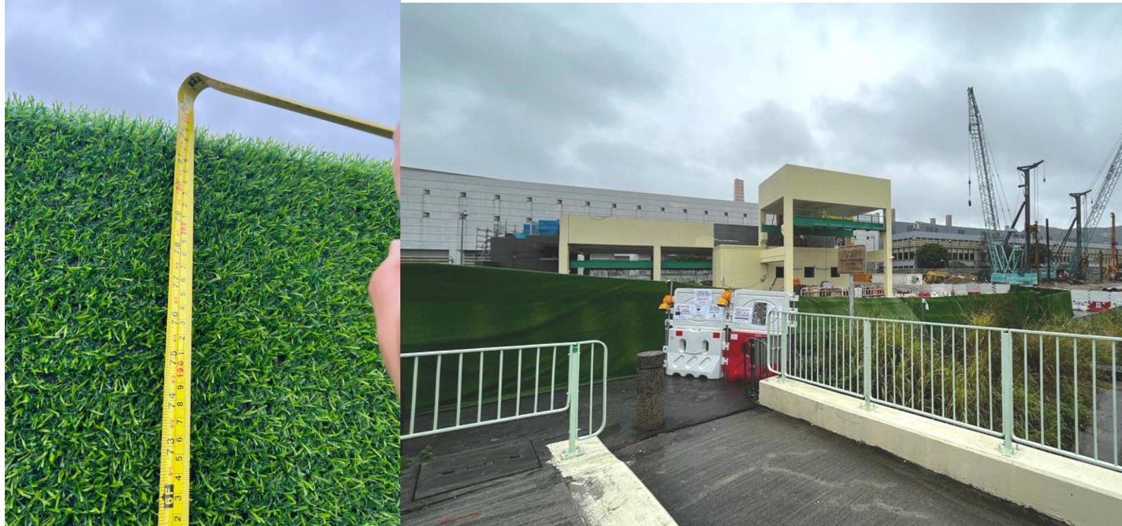
The site barrier fence next to Ng Tung River is completed.
