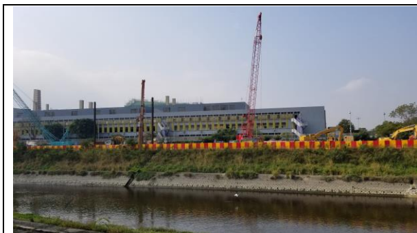
Construction Activities (Ng Tung River) (Non-Project-related, taken on 7 Feb 2022)
