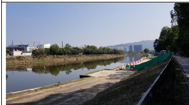
Construction Activities (Sheung Yue River) (Non-project-related, taken on 25 Feb 2022)
