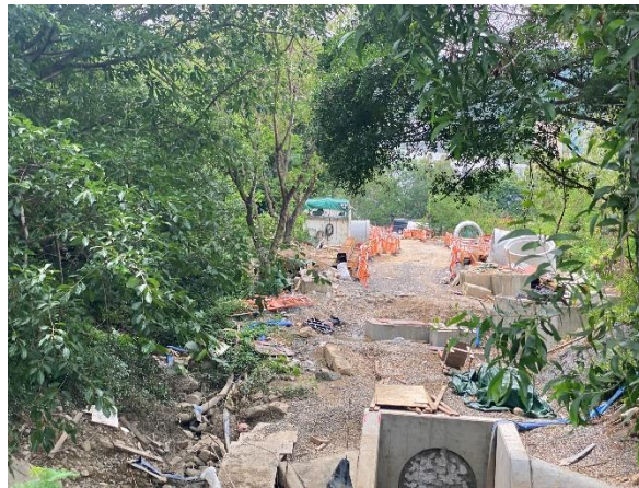
Construction Activities (Sheung Yue River) (Non-project-related, taken on 2 Jun 2022)
