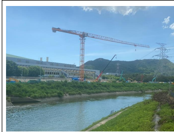
Construction Activities (Ng Tung River) (Non-Project-related, taken on 28 Jun 2022)
