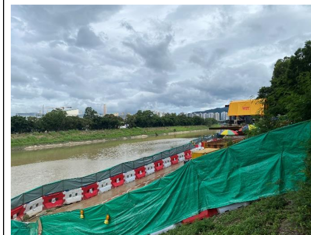
Construction Activities (Sheung Yue River) (Non-project-related, taken on 13 Jun 2022)
