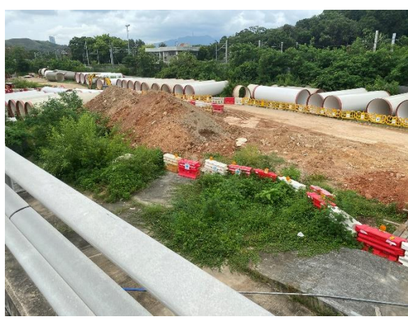
Construction Activities (Sheung Yue River) (Non-project-related, taken on 22 Jun 2022)
