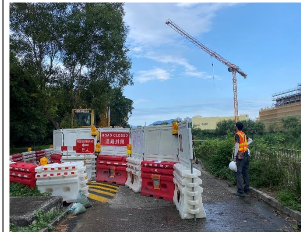
Construction Activities (Ng Tung River) (Non-Project-related, taken on 9 Sep 2022)
