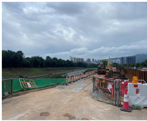
Construction Activities (Sheung Yue River) (Non-project-related, taken on 27 Sep 2022)
