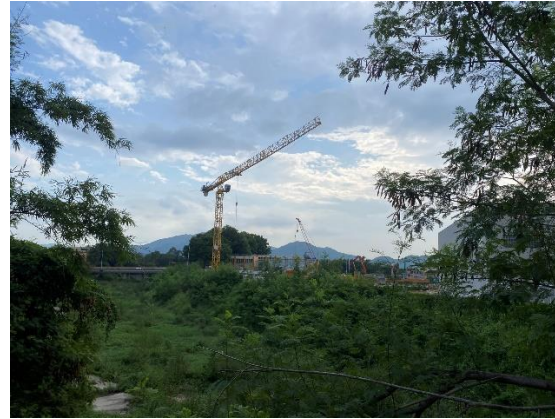
Construction Activities (Shek Sheung River) (Project-related, taken on 9 Sep 2022)
