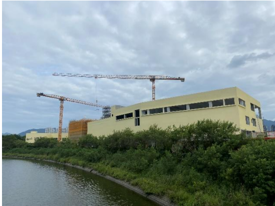
Construction Activities (Ng Tung River) (Project-related, taken on 27 Sep 2022)
