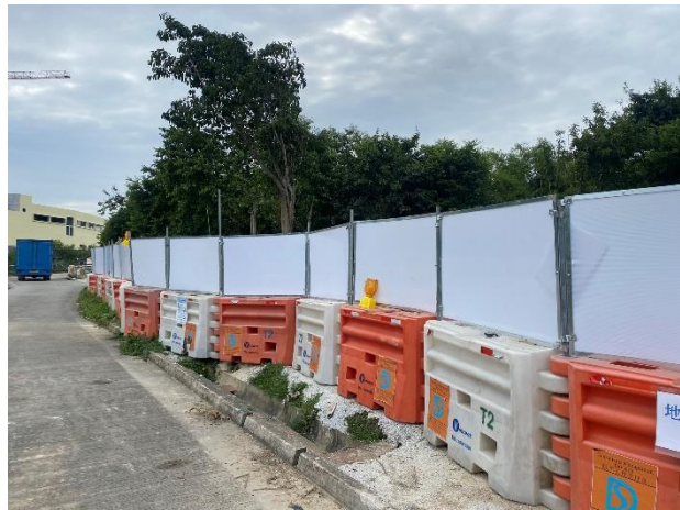
Construction Activities (Ng Tung River) (Non-Project-related, taken on 27 Sep 2022)
