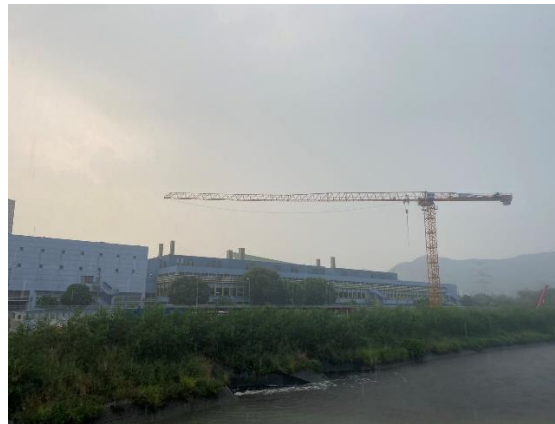
Construction Activities (Ng Tung River) (Non-Project-related, taken on 23 Sep 2022)
