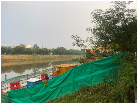
Construction Activities (Sheung Yue River) (Non-project-related, taken on 23 Sep 2022)
