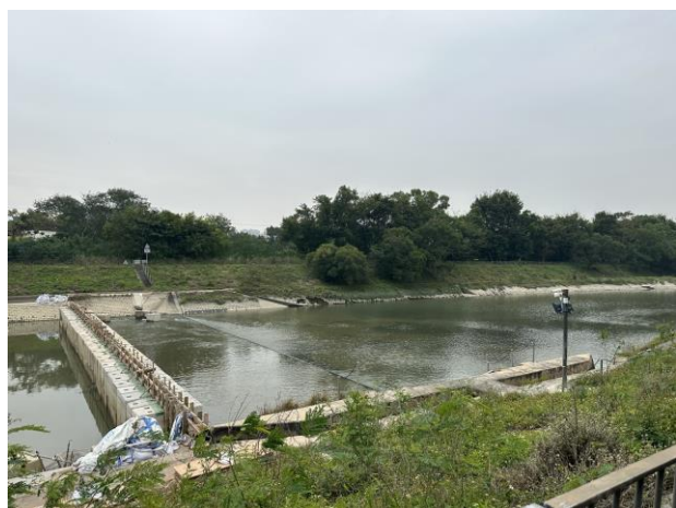
Construction Activities (Ng Tung River) (Non-Project-related, taken on 13 Dec 2022)
