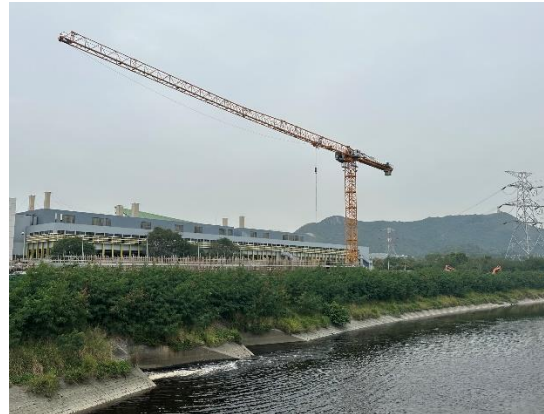
Construction Activities (Ng Tung River) (Non-Project-related, taken on 13 Dec 2022)
