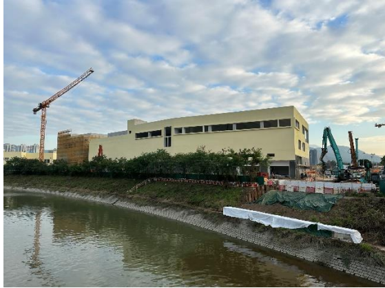
Construction Activities (Ng Tung River) (Project-related, taken on 6 Dec 2022)
