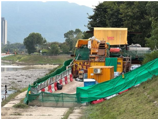
Construction Activities (Sheung Yue River) (Non-project-related, taken on 23 Dec 2022)
