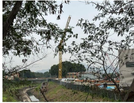
Construction Activities (Shek Sheung River) (Project-related, taken on 13 Dec 2022)
