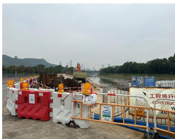
Construction Activities (Sheung Yue River) (Non-project-related, taken on 13 Dec 2022)
