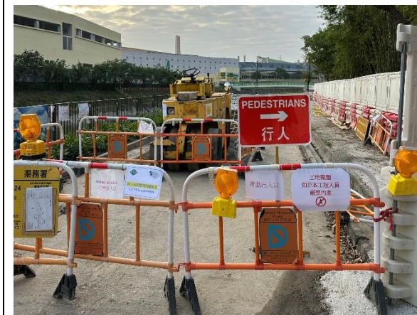
Construction Activities (Ng Tung River) (Non-Project-related, taken on 23 Dec 2022)
