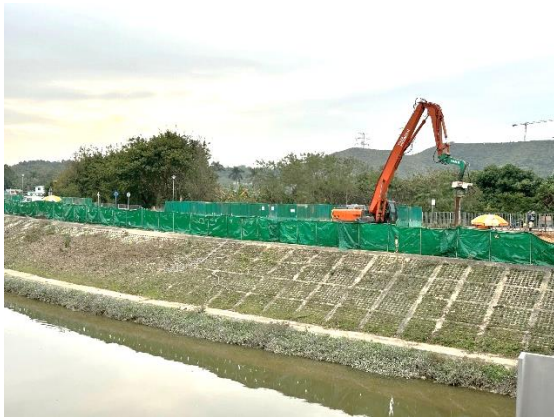
Construction Activities (Sheung Yue River) (Non-project-related, taken on 26 Jan 2023)
