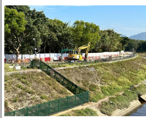
Construction Activities (Ng Tung River) (Non-Project-related, taken on 6 Jan 2023)
