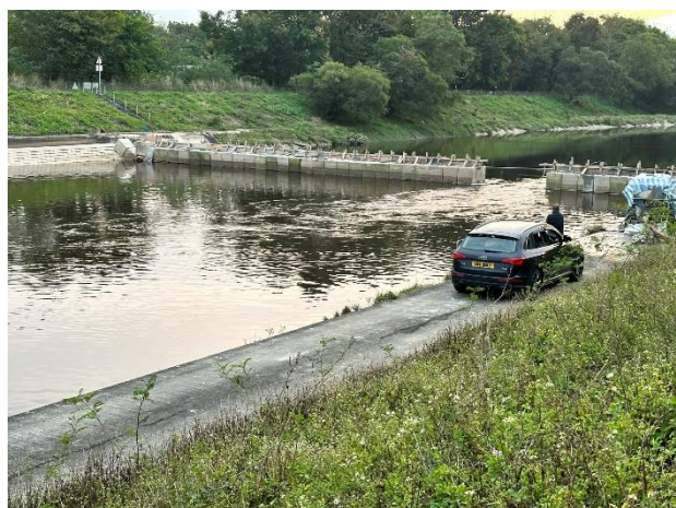
Construction Activities (Ng Tung River) (Non-Project-related, taken on 16 Jan 2023)
