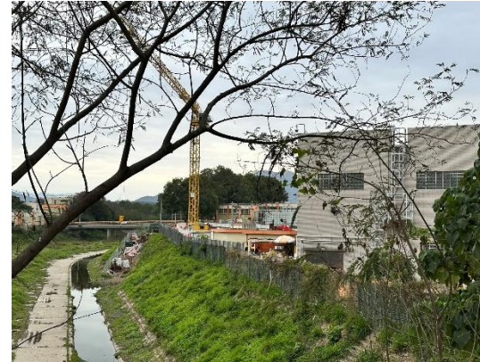
Construction Activities (Shek Sheung River) (Project-related, taken on 26 Jan 2023)
