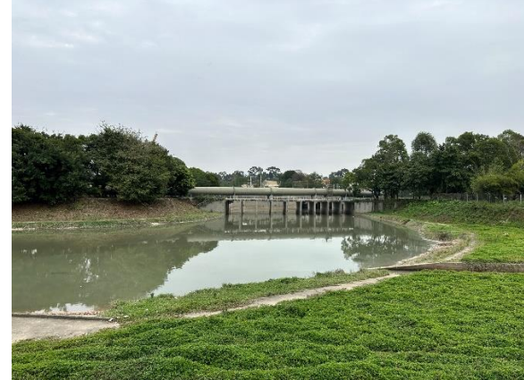
Shek Sheung River – Survey Point 6 (Taken on 16 Jan 2023)
