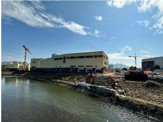
Construction Activities (Ng Tung River) (Project-related, taken on 6 Jan 2023)
