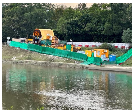
Construction Activities (Sheung Yue River) (Non-project-related, taken on 12 Jan 2023)
