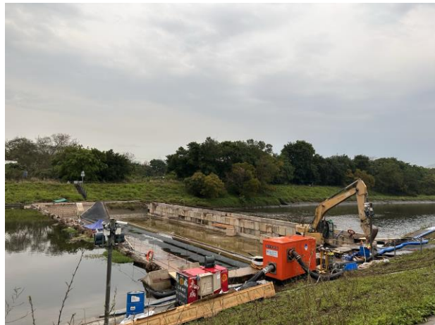
Construction Activities (Ng Tung River) (Non-Project-related, taken on 19 Apr 2023)
