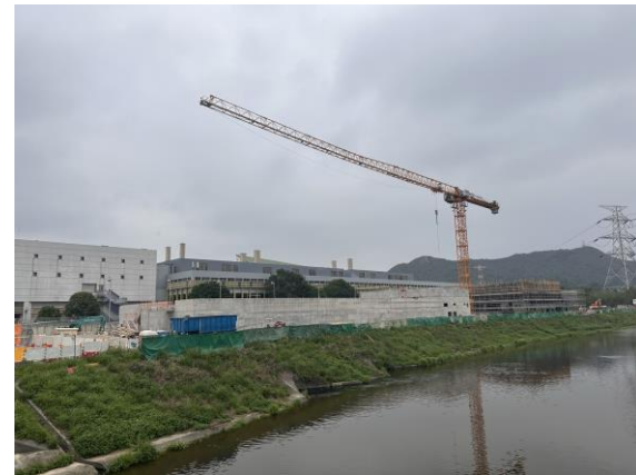
Construction Activities (Ng Tung River) (Non-Project-related, taken on 24 Apr 2023)
