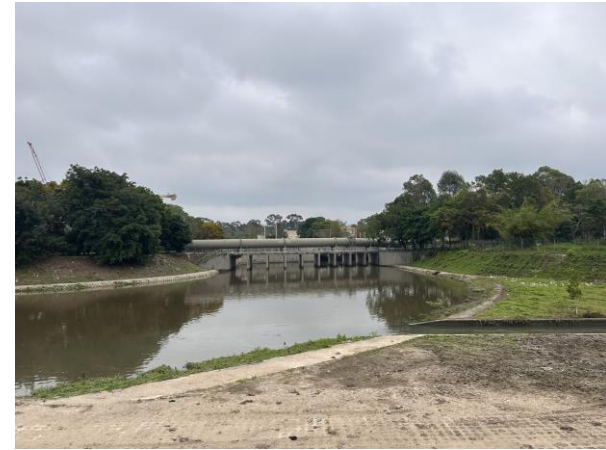
Shek Sheung River – Survey Point 6 (Taken on 24 Apr 2023)
