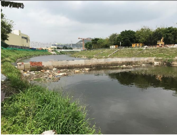
Rubbish and debris trapped between the control station and monitoring station
