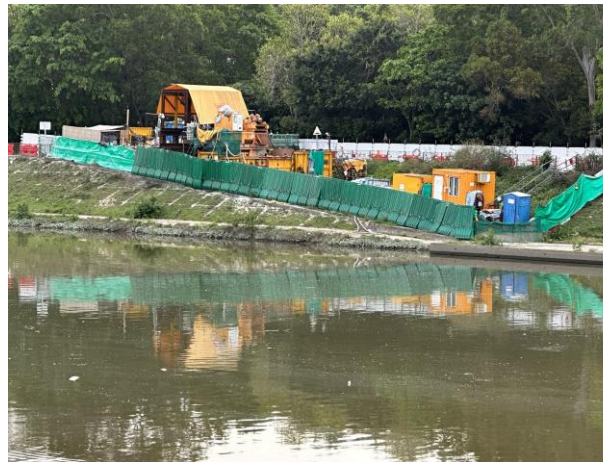
Construction Activities (Sheung Yue River) (Non-project-related, taken on 6 Apr 2023)
