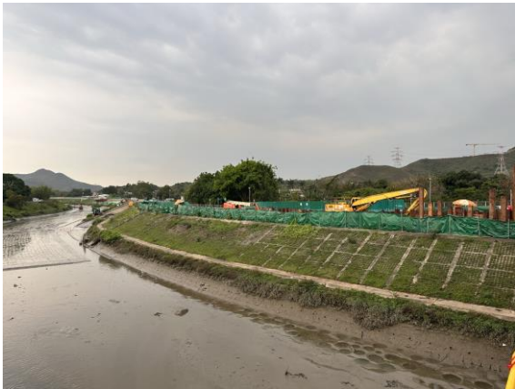
Construction Activities (Sheung Yue River) (Non-project-related, taken on 19 Apr 2023)
