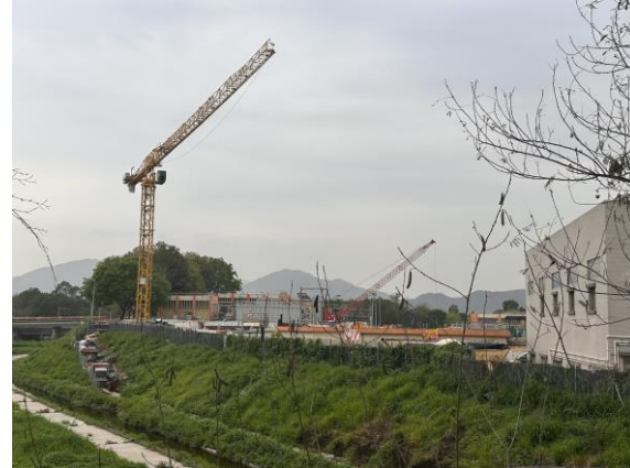
Construction Activities (Shek Sheung River) (Project-related, taken on 6 Apr 2023)
