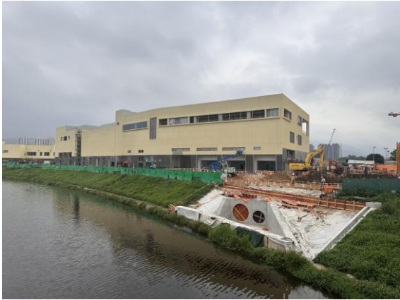
Construction Activities (Ng Tung River) (Project-related, taken on 24 Apr 2023)
