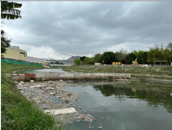
Rubbish and debris trapped between the control station and monitoring station
