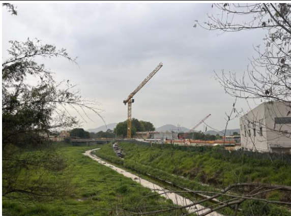
Shek Sheung River - Survey Point 5 (Taken on 6 Apr 2023)
