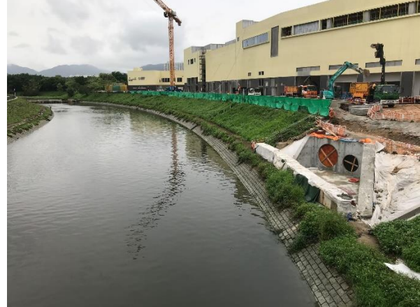
Outfall and the Project Site boundary along Ng Tung River
