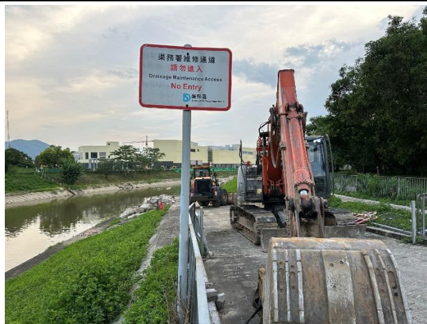
Construction Activities (Ng Tung River) (Non-Project-related, taken on 30 June 2023)
