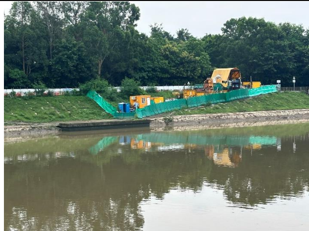
Construction Activities (Sheung Yue River) (Non-project-related, taken on 21 June 2023)
