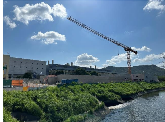
Construction Activities (Ng Tung River) (Non-Project-related, taken on 5 June 2023)
