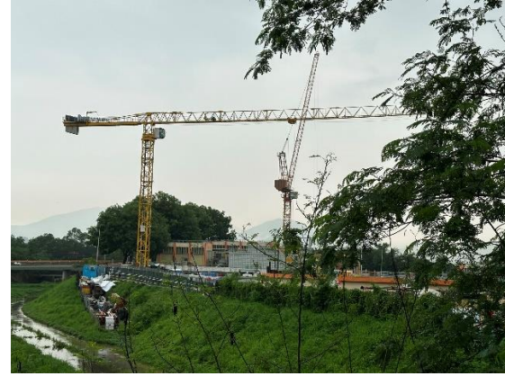
Construction Activities (Shek Sheung River) (Project-related, taken on 15 June 2023)
