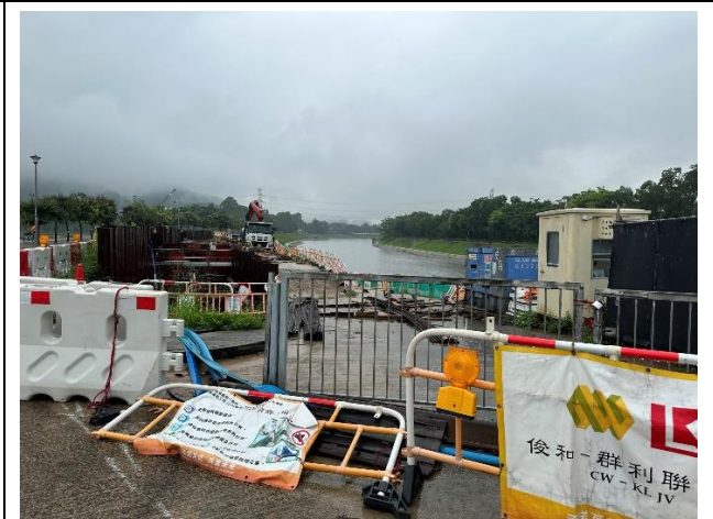
Construction Activities (Sheung Yue River) (Non-project-related, taken on 15 June 2023)
