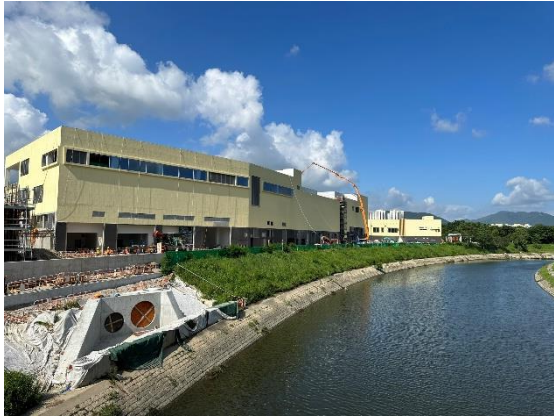
Construction Activities (Ng Tung River) (Project-related, taken on 2 June 2023)
