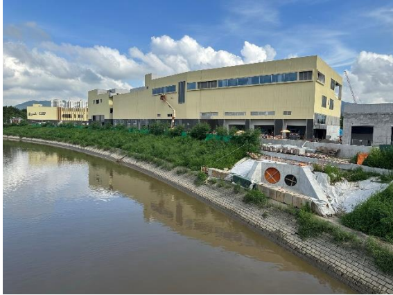
Construction Activities (Ng Tung River) (Project-related, taken on 14 Aug 2023)
