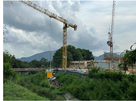
Construction Activities (Shek Sheung River) (Project-related, taken on 30 Aug 2023)
