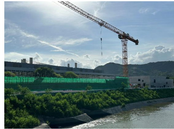
Construction Activities (Ng Tung River) (Non-Project-related, taken on 4 Aug 2023)
