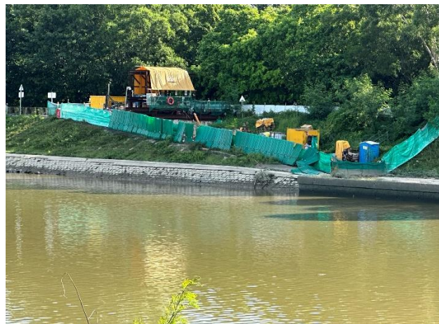
Construction Activities (Sheung Yue River) (Non-project-related, taken on 31 Aug 2023)
