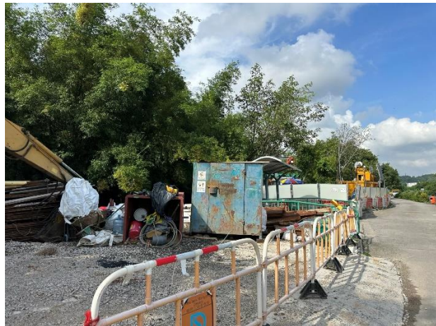
Construction Activities (Ng Tung River) (Non-Project-related, taken on 14 Aug 2023)
