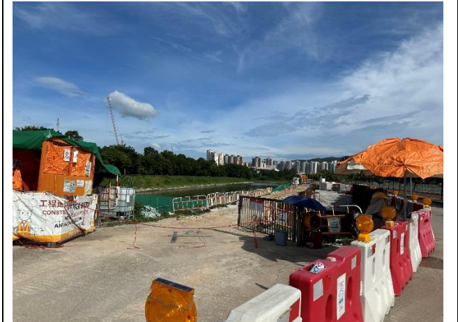
Construction Activities (Sheung Yue River) (Non-project-related, taken on 4 Aug 2023)
