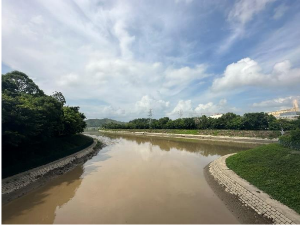
Sheung Yue River – Survey Point 7 (Taken on 14 Aug 2023)
