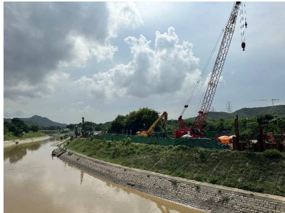
Construction Activities (Sheung Yue River) (Non-project-related, taken on 14 Aug 2023)
