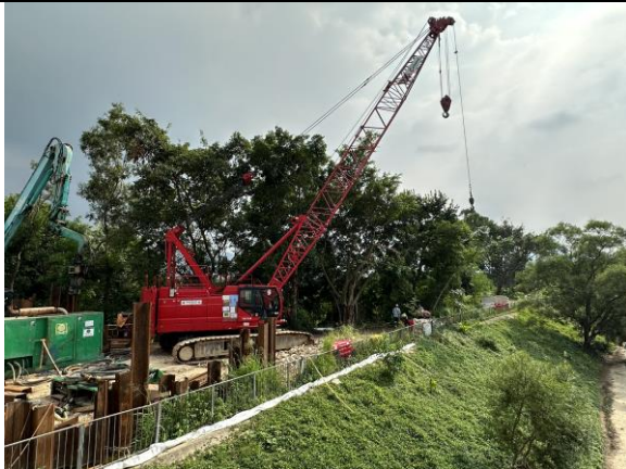
Construction Activities (Sheung Yue River) (Non-project-related, taken on 12 Oct 2023)
