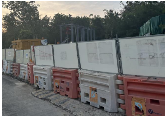
Construction Activities (Ng Tung River) (Non-Project-related, taken on 16 Oct 2023)
