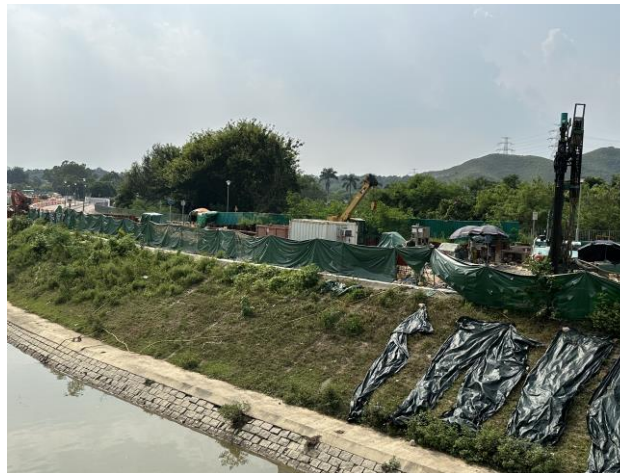
Construction Activities (Sheung Yue River) (Non-project-related, taken on 12 Oct 2023)
