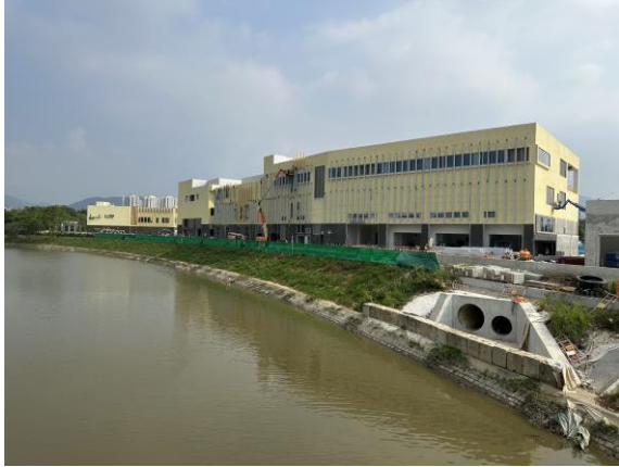
Construction Activities (Ng Tung River) (Project-related, taken on 3 Oct 2023)
