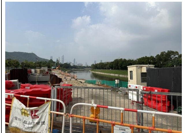
Construction Activities (Sheung Yue River) (Non-project-related, taken on 12 Oct 2023)
