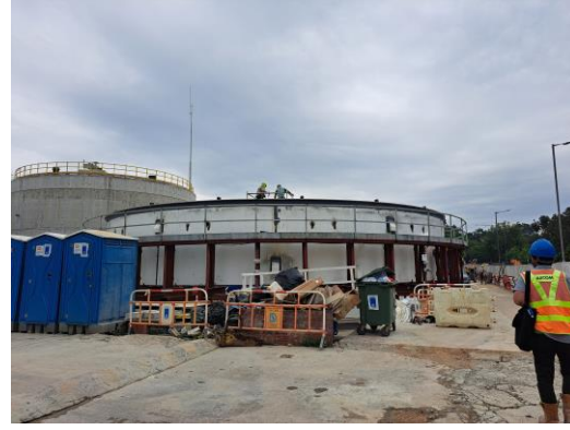
Bio Gas Tank
