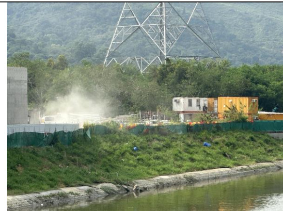
Construction Activities (Ng Tung River) (Non-Project-related, taken on 12 Oct 2023)
