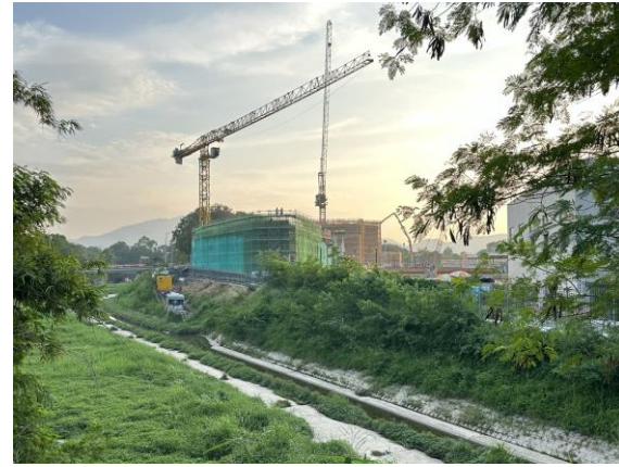
Construction Activities (Shek Sheung River) (Project-related, taken on 16 Oct 2023)
