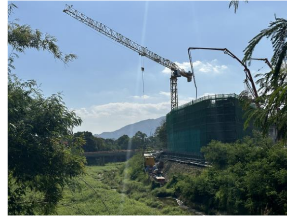
Construction Activities (Shek Sheung River) (Project-related, taken on 21 Nov 2023)
