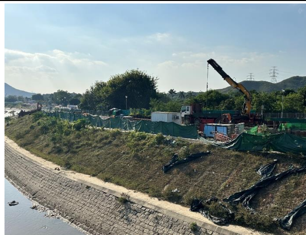
Construction Activities (Sheung Yue River) (Non-project-related, taken on 21 Nov 2023)
