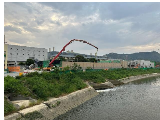
Construction Activities (Ng Tung River) (Non-Project-related, taken on 10 Nov 2023)
