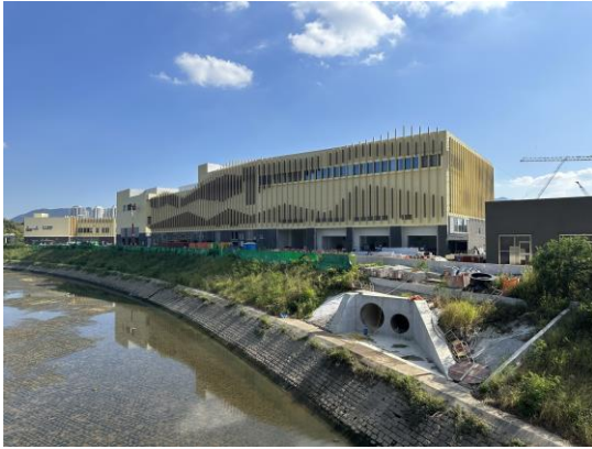
Construction Activities (Ng Tung River) (Project-related, taken on 15 Nov 2023)
