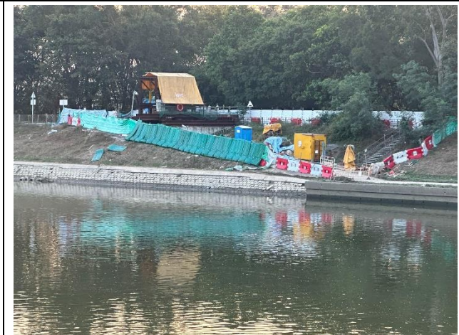
Construction Activities (Sheung Yue River) (Non-project-related, taken on 29 Nov 2023)
