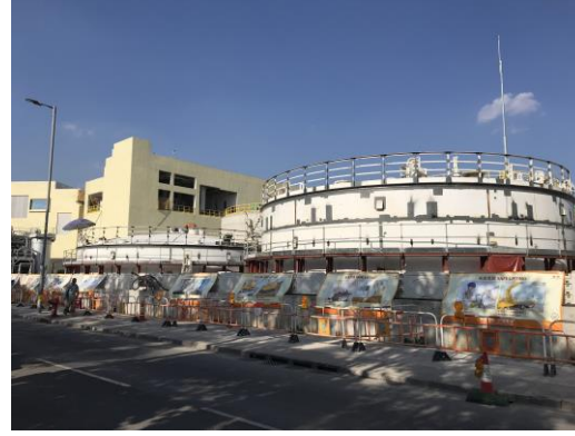
Bio Gas Tank
