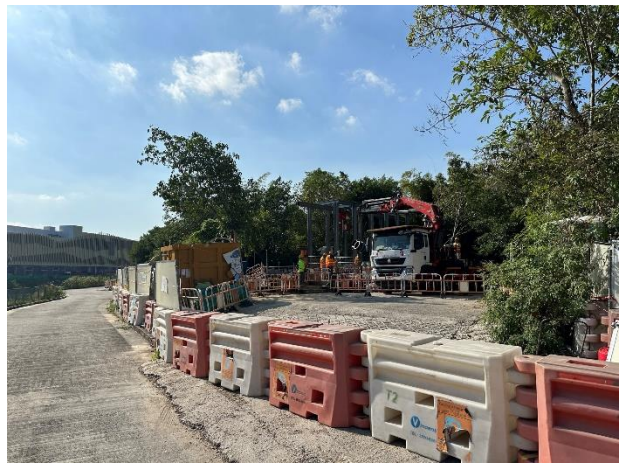
Construction Activities (Ng Tung River) (Non-Project-related, taken on 15 Nov 2023)
