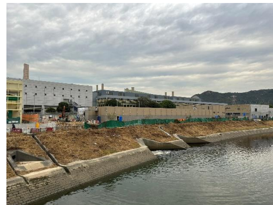
Construction Activities (Ng Tung River) (Non-Project-related, taken on 25 Jan 2024)
