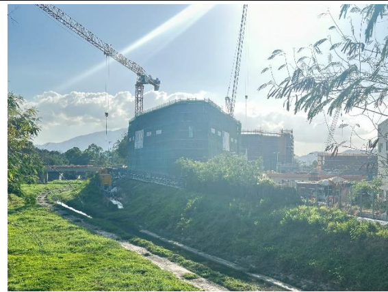
Construction Activities (Shek Sheung River) (Project-related, taken on 12 Jan 2024)
