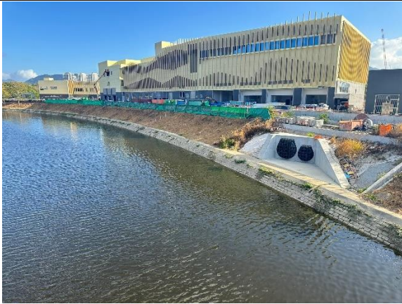
Construction Activities (Ng Tung River) (Project-related, taken on 5 Jan 2024)
