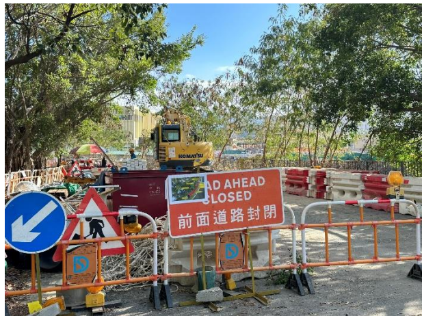
Construction Activities (Ng Tung River) (Non-Project-related, taken on 12 Jan 2023)
