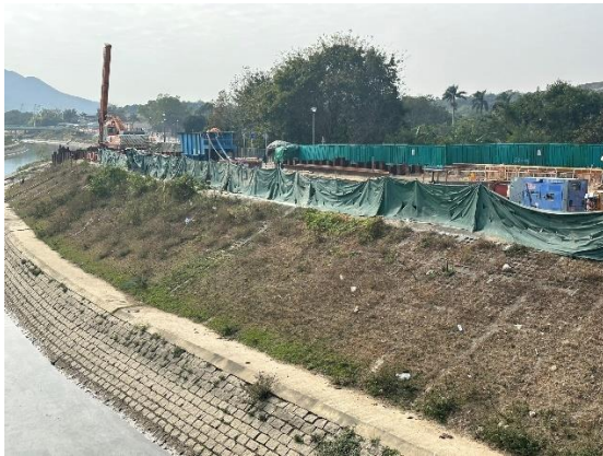
Construction Activities (Sheung Yue River) (Non-project-related, taken on 31 Jan 2024)
