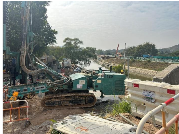
Construction Activities (Sheung Yue River) (Non-project-related, taken on 25 Jan 2024)
