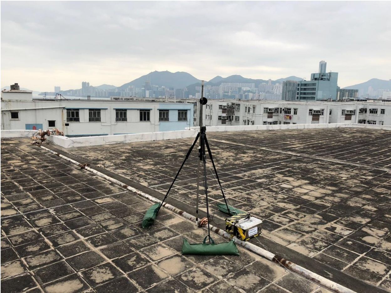
Noise Monitoring Station E-N21a – Block B, Merit Industrial Centre Rooftop
