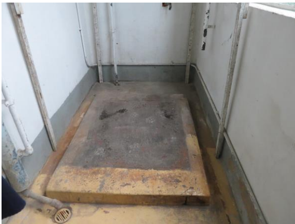
Figure 5.1 Demolition of incinerator was completed
