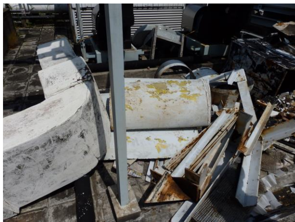
Figure 4.2 Steel framework and outer steel shell were cut to smaller pieces
