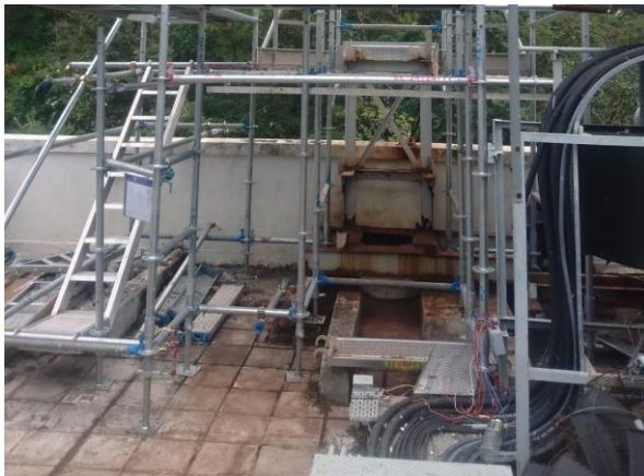
Figure 5.5 View of Rooftop
