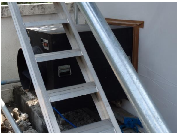
Figure 3.20 Air mover for the works area at Rooftop
