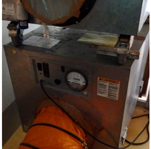
Figure 3.25 Air movers for the works area at 5/F
