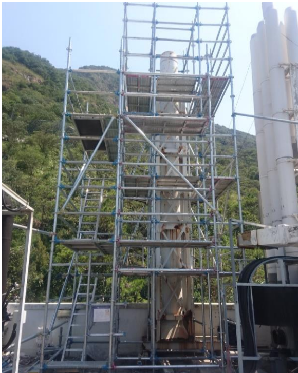
Figure 3.14 Scaffold at the Rooftop
