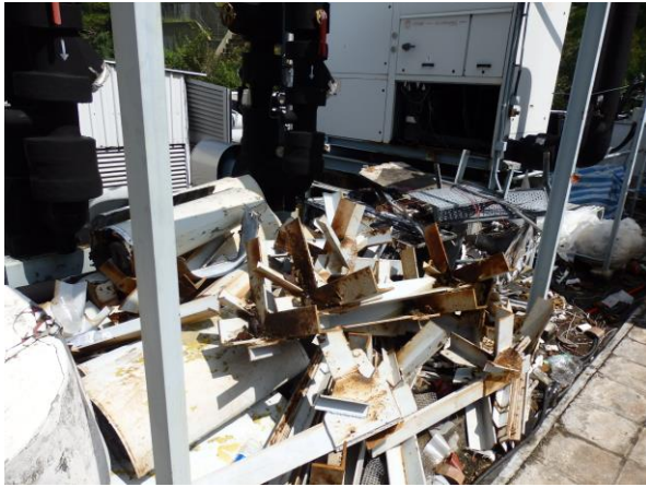
Figure 4.3 Steel framework and outer steel shell were cut to smaller pieces
