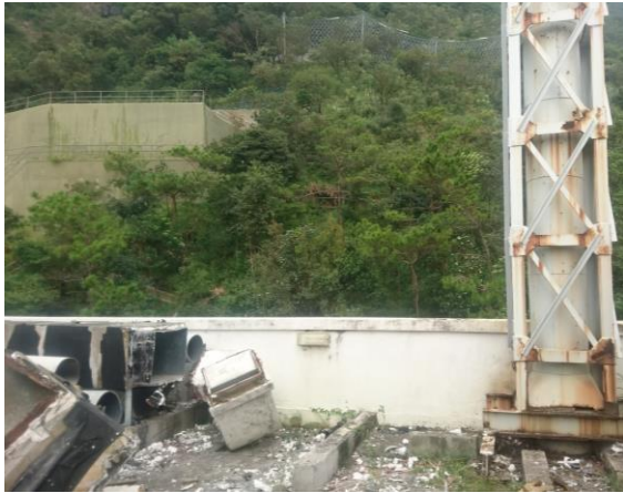
Figure 3.9 Ductworks in front of the chimney of the incinerator were removed
