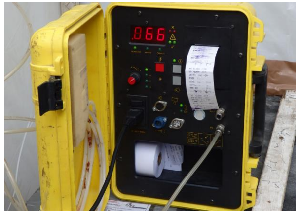
Figure 3.16 Smoke test was conducted for the containment at Rooftop
