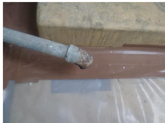
Figure 3.13 Sealed drain
