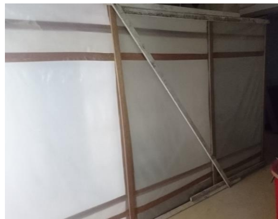
Figure 3.11 Three-compartment decontamination unit for entry and exit into the works area
