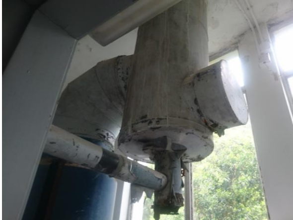
Figure 3.3 Chimney of the Incinerator
