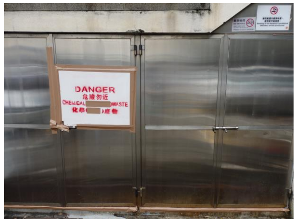
Figure 3.29 Lock is provided for the refuse storage area
