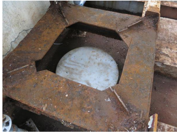
Figure 5.4 Demolition of the associated chimney of the incinerator was completed
