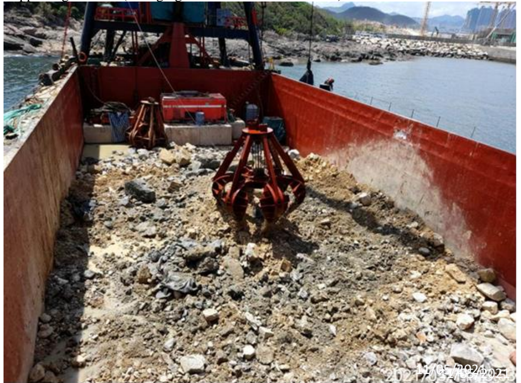
Supporting Photo 5 (Dredging Activities at Outfall Shaft)
